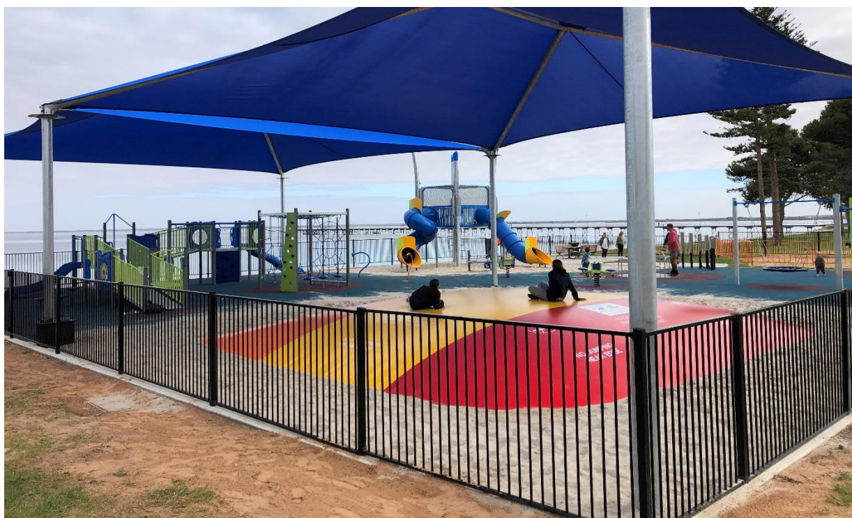
Ceduna Foreshore Playground recently constructed in 2021 is one of many Open Spaces that are maintained by Council.
